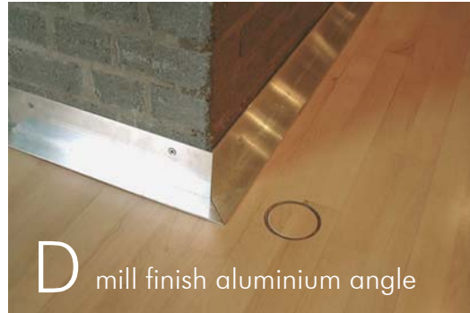
Mill finish aluminium angle skirting 50 x 50 x 3mm, or 75 x 50 x 3mm profiles
