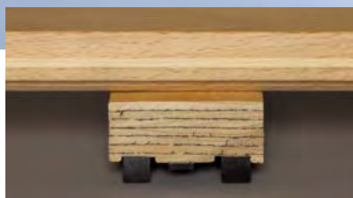
Rubber strips in unloaded position.
