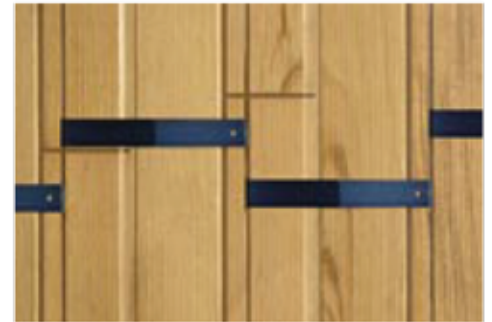
The clips hold the boards together - on the back of the boards.
